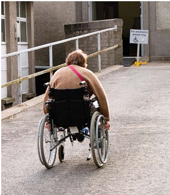
Less force is needed to push a load up a ramp than to push it straight up
